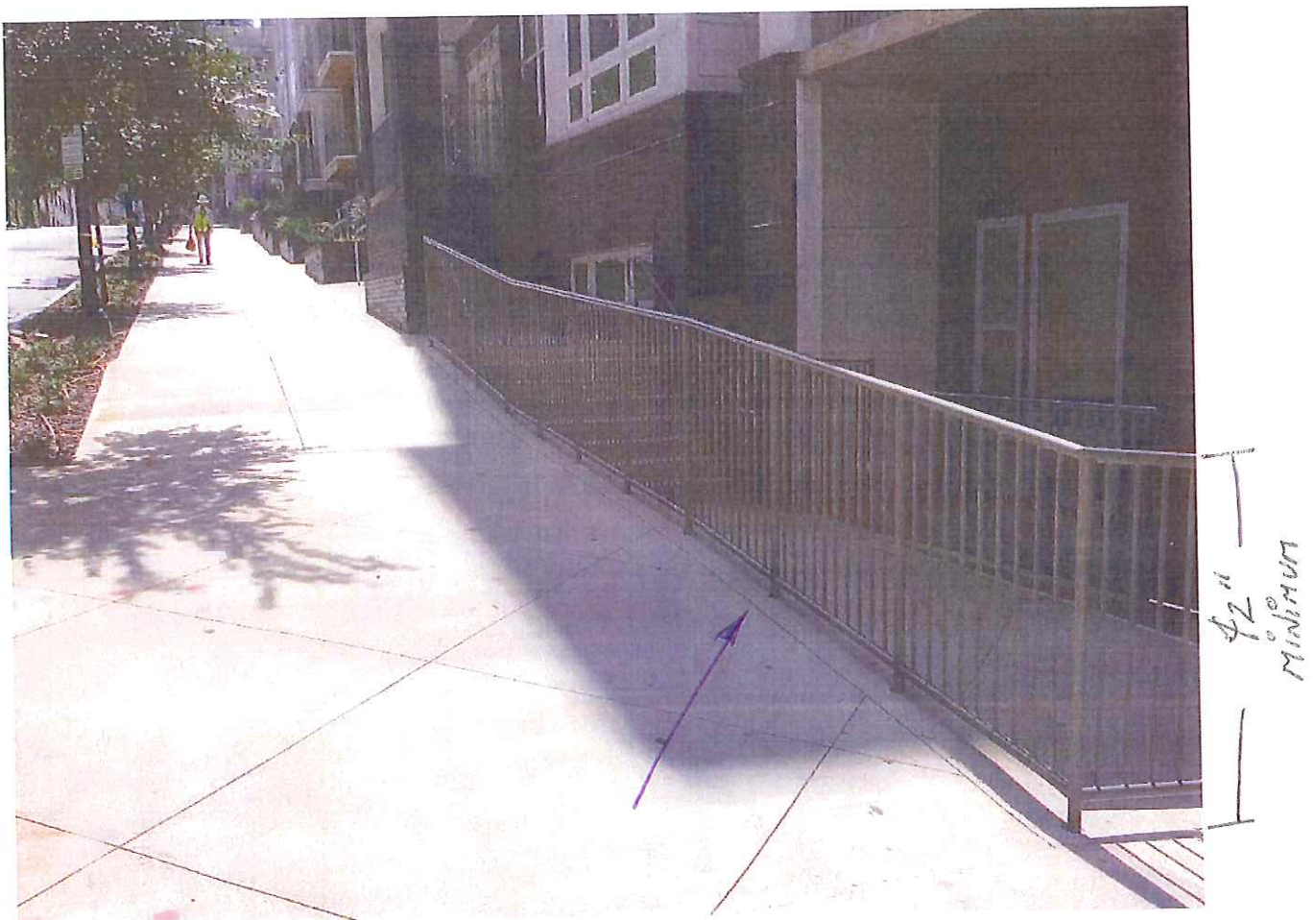
Figure 4.13. Pedestrian Safety Railing, Midtown, Atlanta, Georgia
